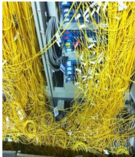
Figure 1 Paper labeling of optical fibers
